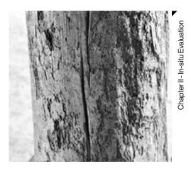
▲ Fig. 44/ Column attacked by beetles. Source: Wang, s.: damage classification to historical wooden structures: a preliminary survey and recommendation for Dong minority drum towers, int. Arch. Photogramm. Remote sens. Spatial inf. Sci., xlvi-m-1-2021, 821–827, 2021 https://doi.org/10.5194/isprs-archives-XLVI-M-1-2021-821-2021
