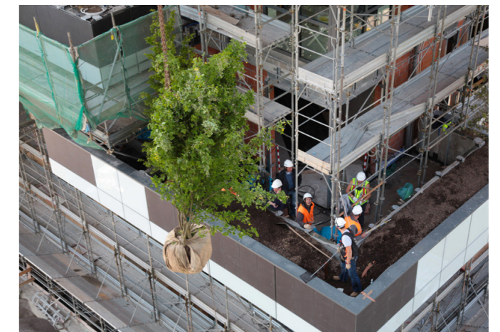
Fig. 65: installation of plants. Source: marco garofalo.
