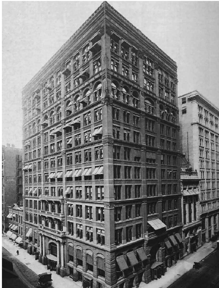
Fig. 03: Home Insurance Building, Chicago, 1884.
