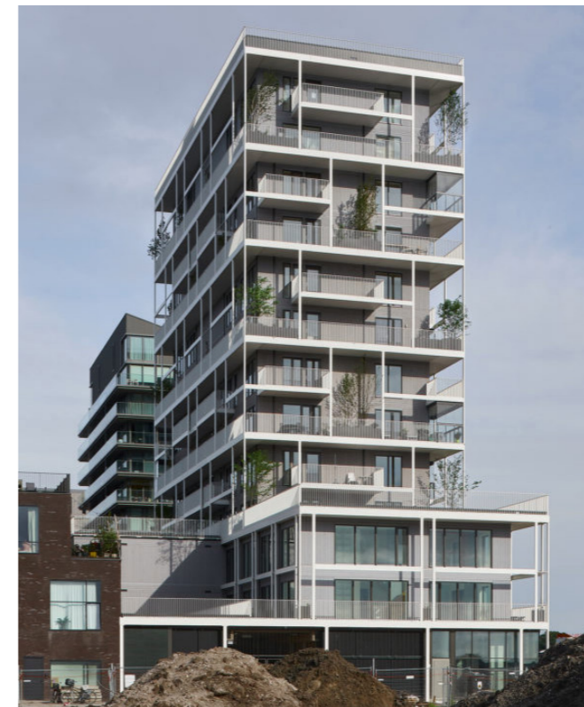
Fig. 58: Stories, Amsterdam, under construction. Source: https://olafgipsen.com/projects/residential-building-bsh/
