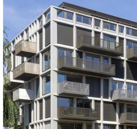
Fig. 52: Facade of the building. Source: https://architectenweb.nl/nieuws/artikel.aspx?ID=46023#photoid=315607
