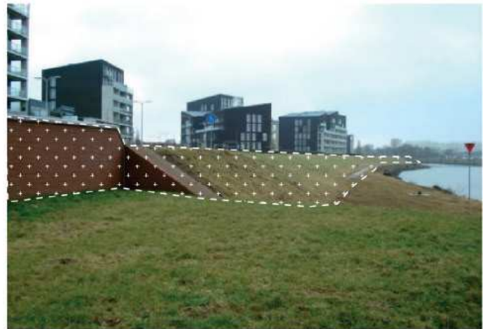
The flood wall can be elevated Figure 24:
