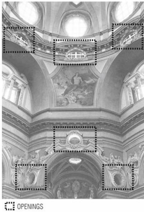
FIGURE 51- PLACEMENT OF THE OPENINGS IN LOCATION OF CRONICE RING AND PLACES THAT SEEM TO NEED THE MAXIMUM REINFORCEMENT - SAN LORENZO – TORINO
