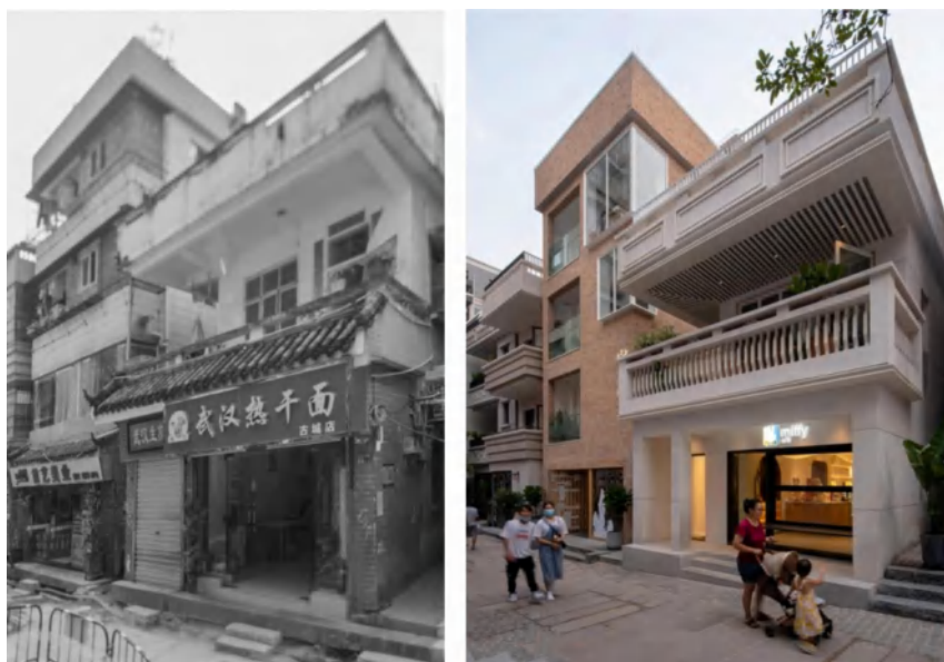
Figure 2-5 Facade Renovation of Nantou Ancient City Buildings Source: Shenzhen Bowan Design ( http://www.szbowan.com/ )
