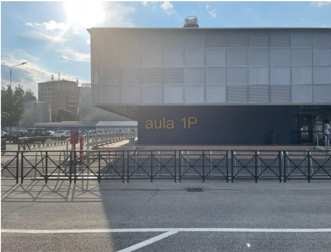
Figure 8: Aule 1P façade view.
