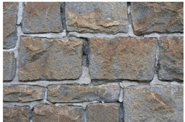
(Fig.49) “opera incerta” local materials used in the building of Asilo Nido Adriano, (Gianotto et al., 2015)
