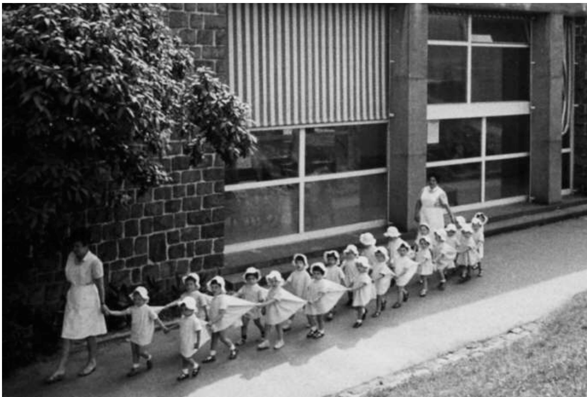
(Fig.2) of the east facade of the Borgo Olivetti nursery school, 1950s, Olivetti historical archive
