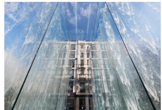
Fig.7, Water as a biophilic attribute used in building Apple's Piazza Liberty Store, Milan (Italy), by Foster p Partners, built in 2018
