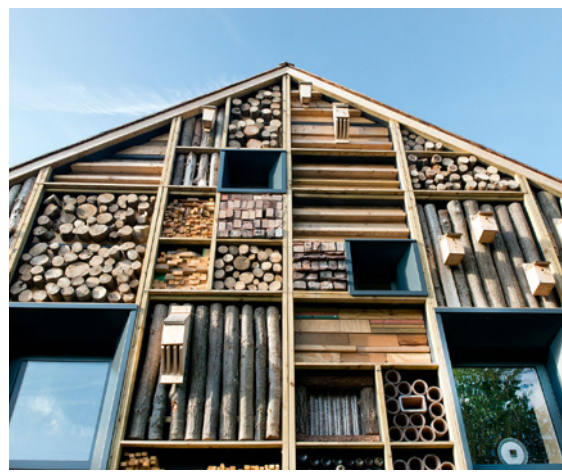
Fig.8 Animals as a biophilic attribute used in building Mellor Primary School, Stockport (UK), by Sarah Wigglesworth Architects, built in 2015
