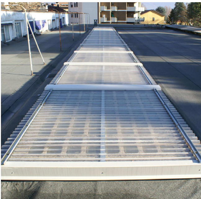
(Fig.52) Skylight above the gallery . (Gianotto et al., 2015)
