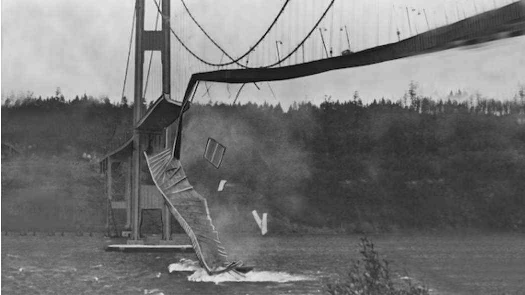
Figure 22: Tacoma Narrows Bridge after flutter phenomenon [20]
