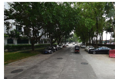
Hujing 1st Street
