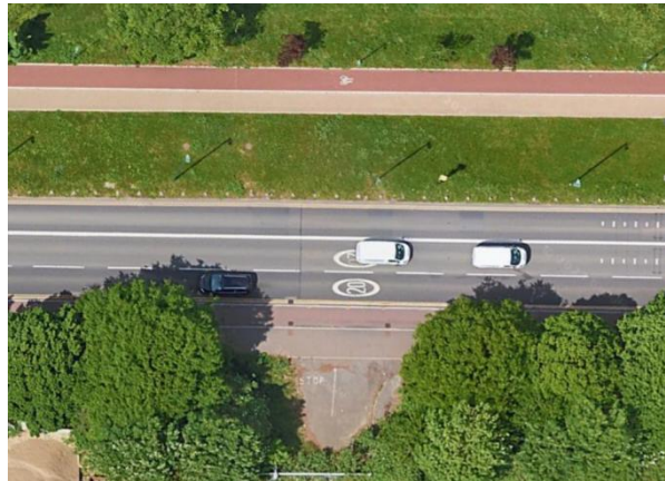
Figure 3-6: Cycling lanes on Lea Bridge Road
