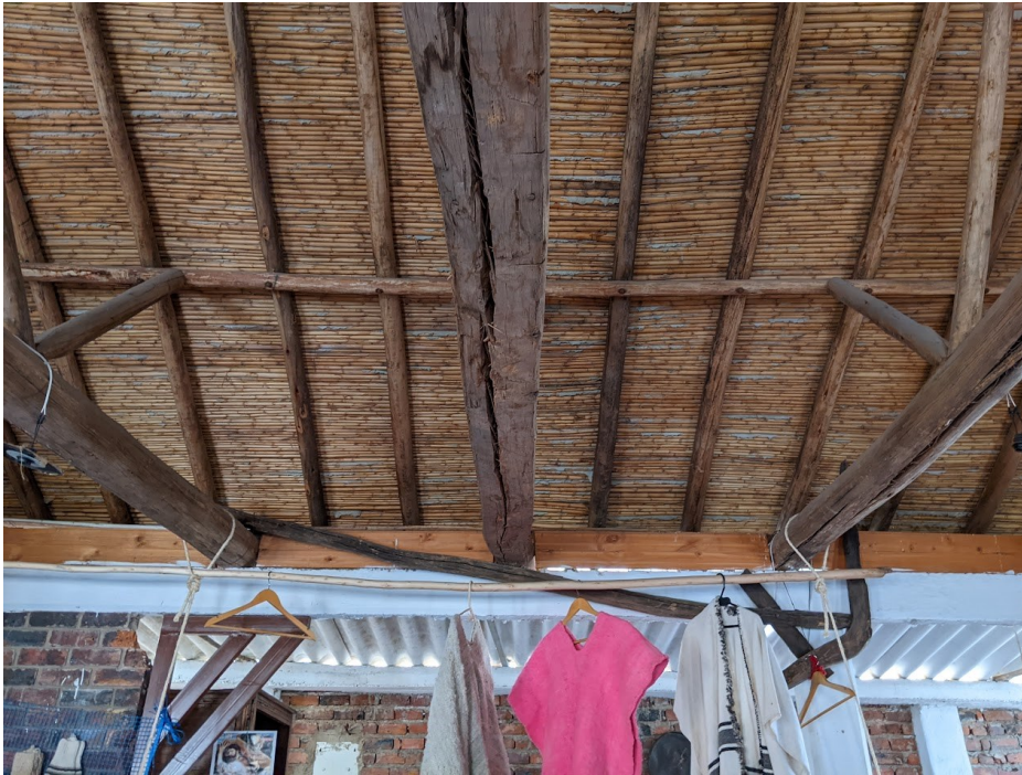
Figure 40: Photography - Presence of "Esterilla" ceiling in traditional rural construction - Nobsa, Boyacá, 2022.
