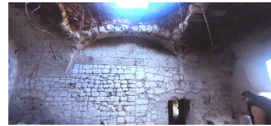
1) BUCKLED CEILING WITH ROOTS OF VEGETATION ABOVE GROWING THROUGH THE VOID
