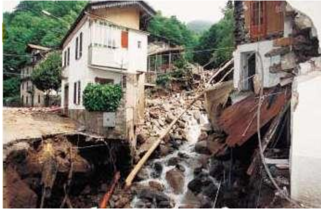
Figure 10. Partial destruction of a residential building in High Cervo Valley. (13)
