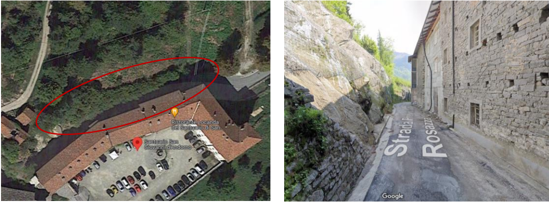
Figure 101. Top view and street view of the terrain slope from Google Maps.
