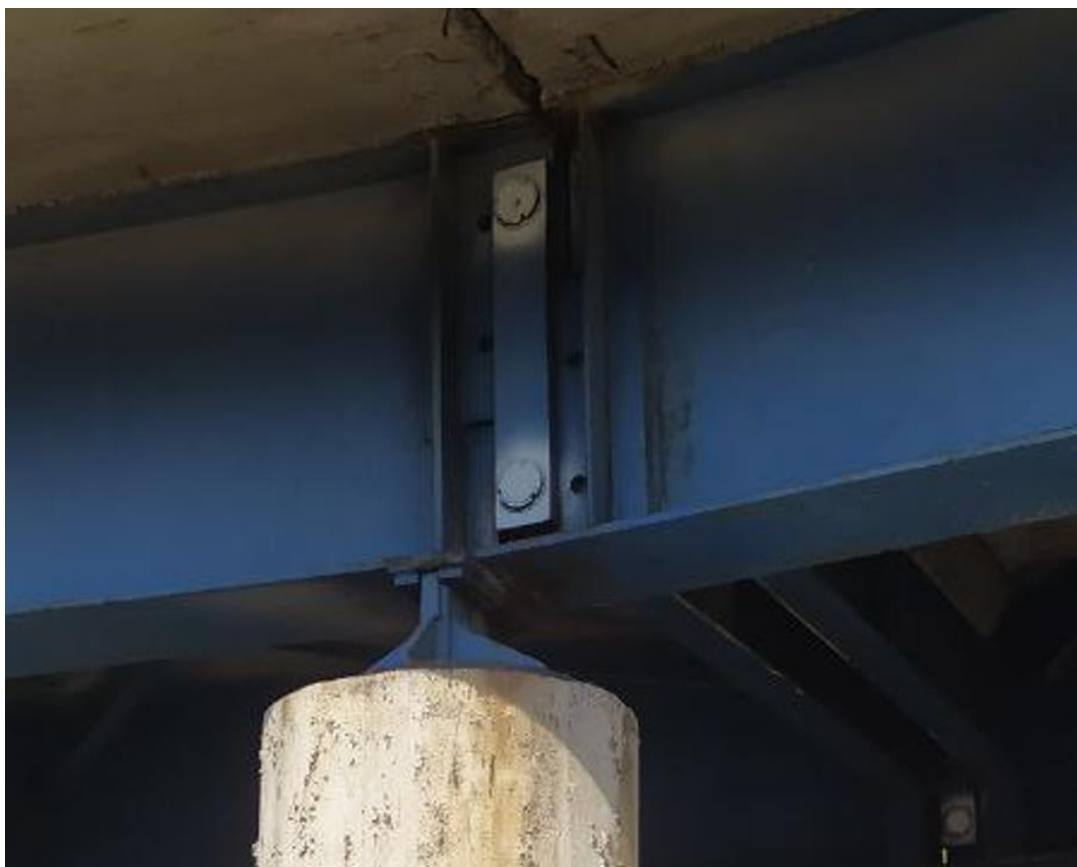
Figure 7-10: Longitudinal beam - pile connection
