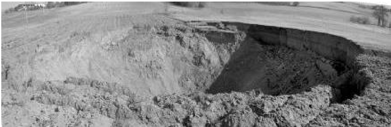
Figure 8 shows the sinkhole that has appeared in the Moncalvo gypsum quarry region. (Geo-surveying for safe underground mining in gypsum deposit in Monferrato basin (Italy) / BONETTO S; FORNARO M; OGGERI C.. - (2006), pp. 382-387. ((Intervento presentato al convegno MPES2006 tenutosi a Turin nel 20-22 Sept.2006) [25].
