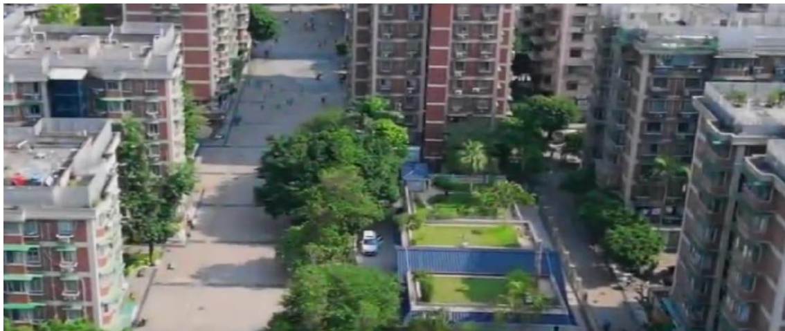
Figure 5-15. Entrance to pedestrian street
