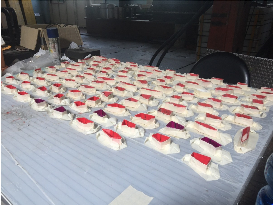
Figure 66: Formworks assembled and positioned for cast operations
