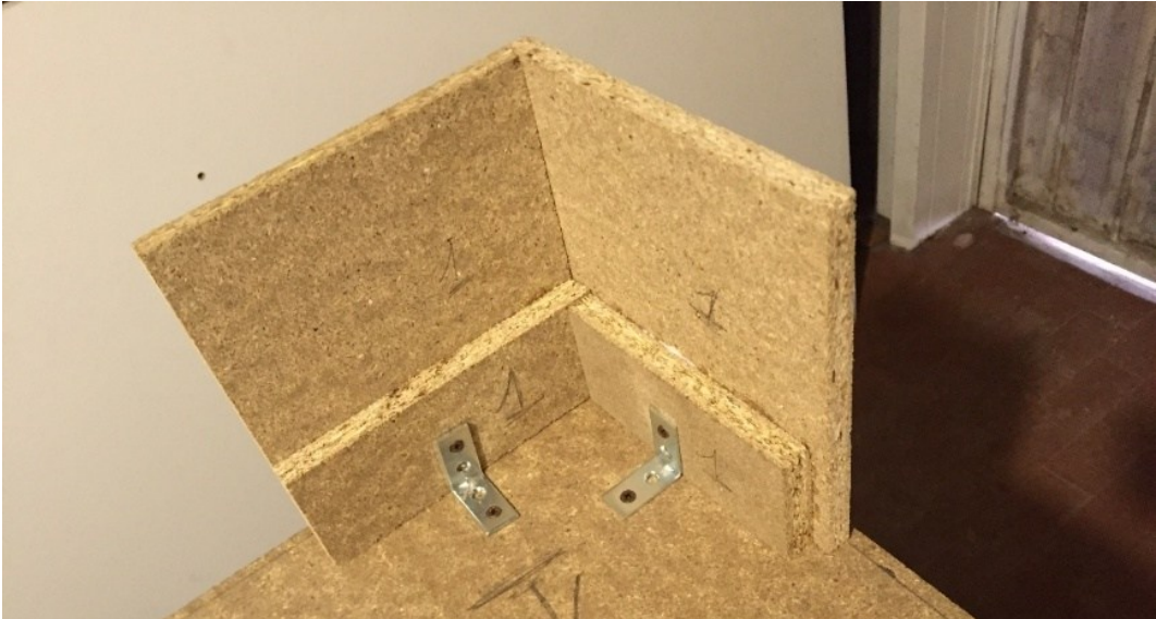
Figure 75: Base constraint detail
