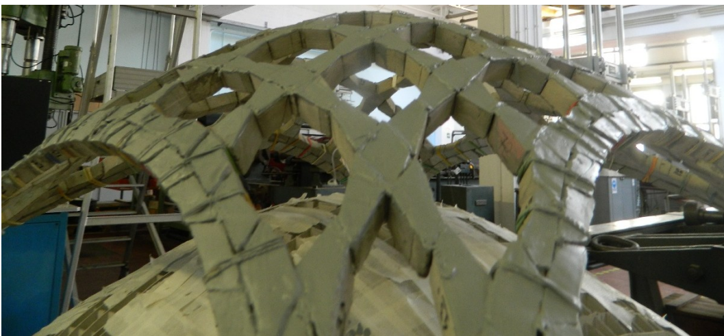
Figure 93: The ended prototype during falsework removal phase – picture 3
