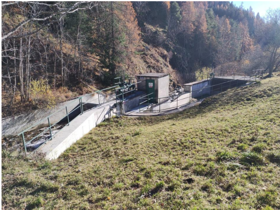
Figure 15: Diversion of the Graines River for the Isollaz Power Plant
