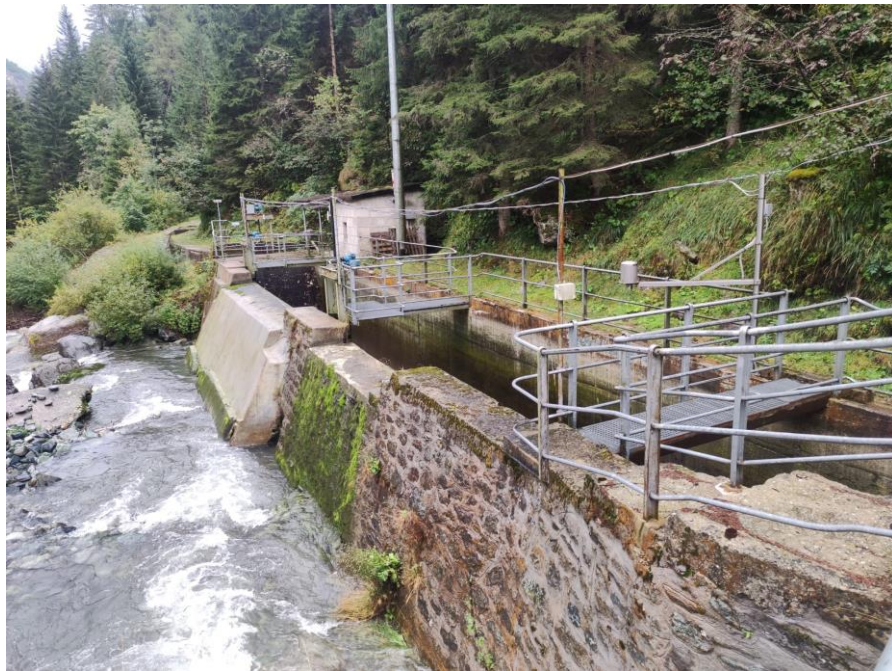
Figure 13: Diversion of the Ayasse River for the Hone Power Plant
