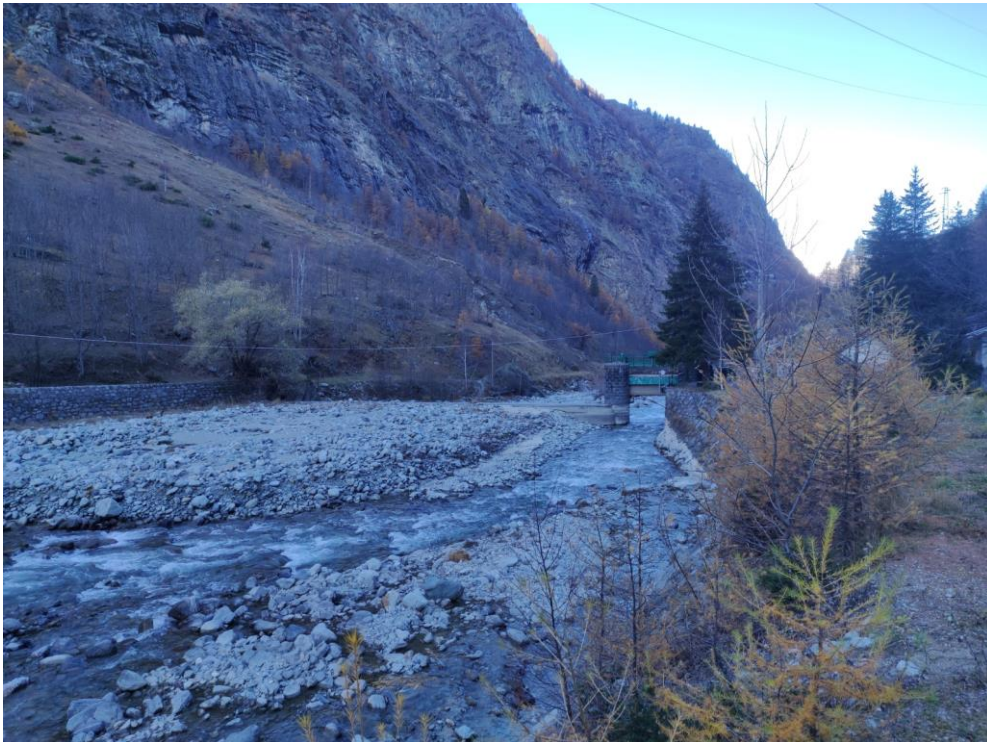
Figure 17: Diversion of the Savara River for the Chavonne Power Plant
