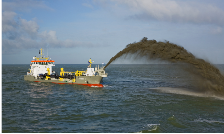
Figure 8: Hydraulic Filling Rainbowing technique example: a Trailing suction hopper dredger pumping sand [25].
