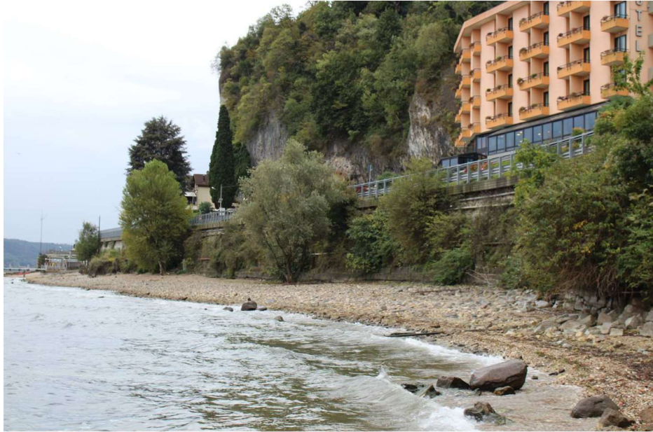
Figure 23. View of the retaining wall
