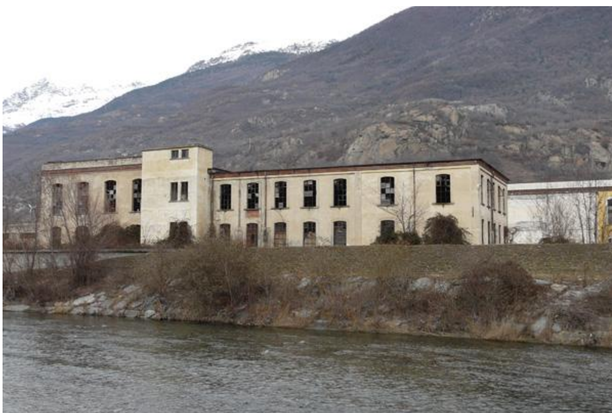
Gennaio 2013, Borgone, The former cotton mill south facade on the Dora Riparia river
