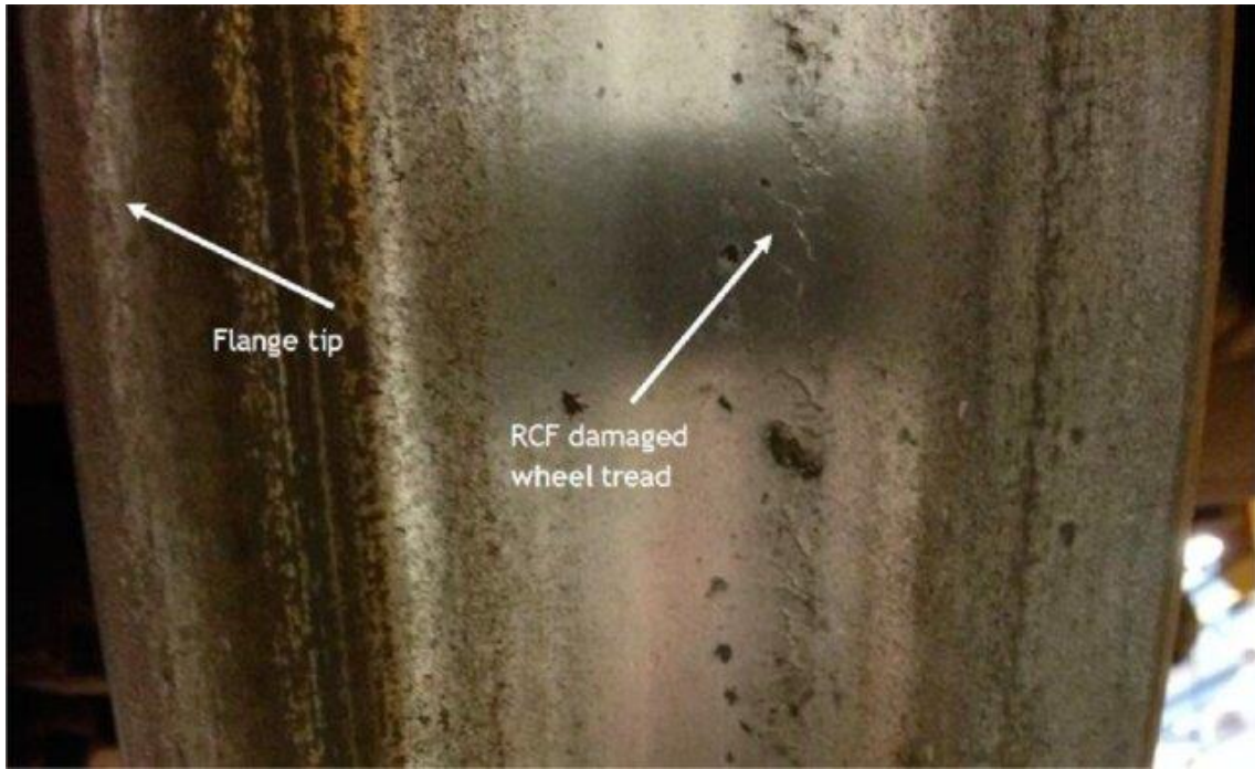
Figure 2.1: Wheel tread with RCF damage highlighted. Taken from: “Enhancing rail infra durability through freight bogie design” [22].
