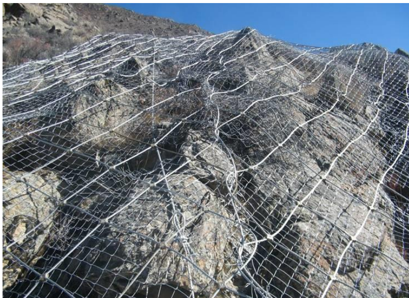
Figure 60 - An example of an active netting system (from Walcoom website).
