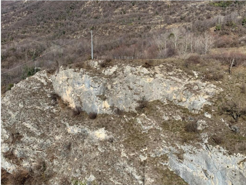
Figure 24 - Overall recovery of the wall in the hydrographic right (blocks L, M, U, V).
