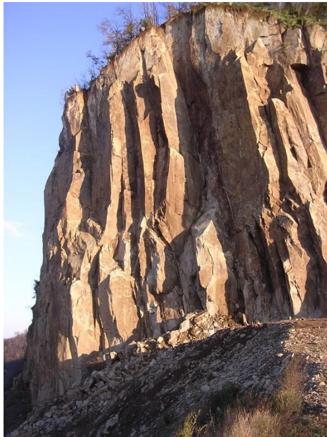
Figure 5 - Example with slabs are clearly visible.
