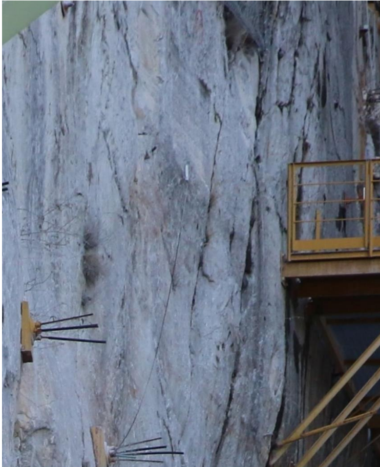
Figure 67 - Tiltmeter in vertical wall in underground marble quarry (Oggeri).
