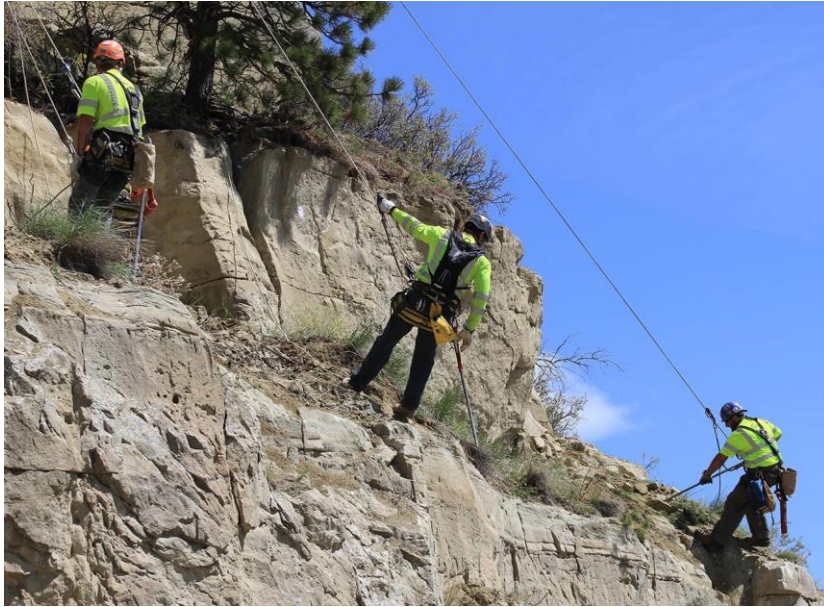
Figure 59 - Three operators by performing rock scaling (from GeoStabilization International).
