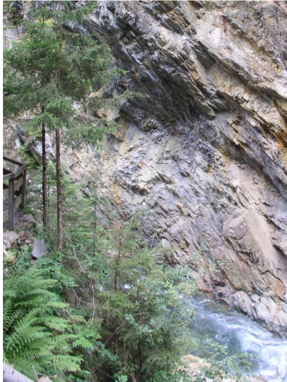
Figure 9 – On the left, path with handrail near the Gorge de la Diosaz (Oggeri C.).
