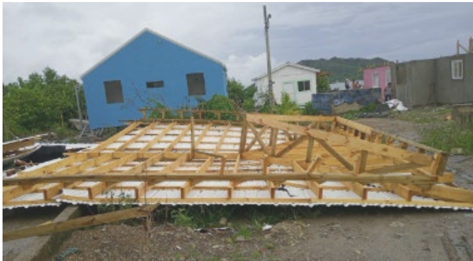
Fig. 168. Roof damage due to a hurricane. Source: Findeter, (2022).
