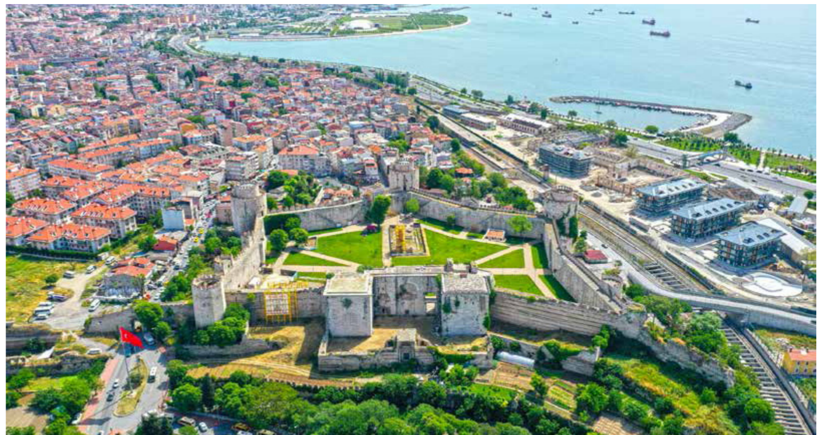
Yedikule Fortress Museum with ongoing restoration project ( https://www.aa.com.tr/tr/kultur-sanat/zamana-meydan-okuyan-yedikule-hisarinda-restorasyon-calismalari-suruyor/2259211 ).
