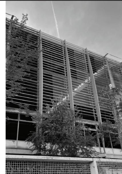
Figure 141: Renovated shading elements, 2023.
