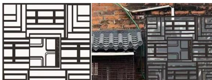
Figure 5-7 Air Conditioner Outdoor Unit Renovation
