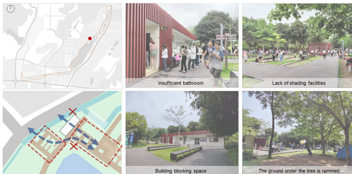
Figure 6-30 Existing Problems in the Central Plaza (self-drawn)
