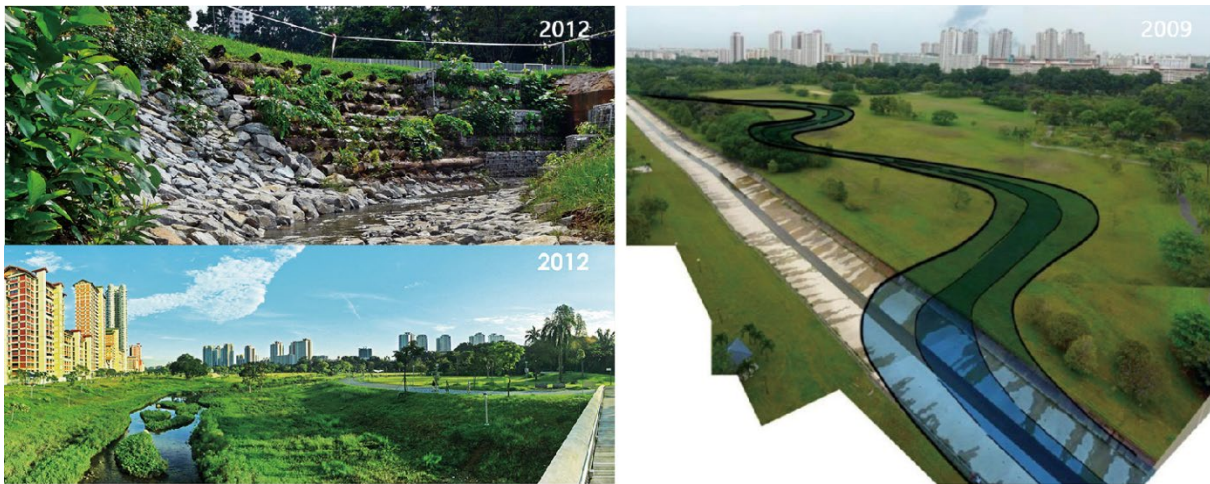
Figure3- 2 Restoring natural curves while preventing soil erosion
