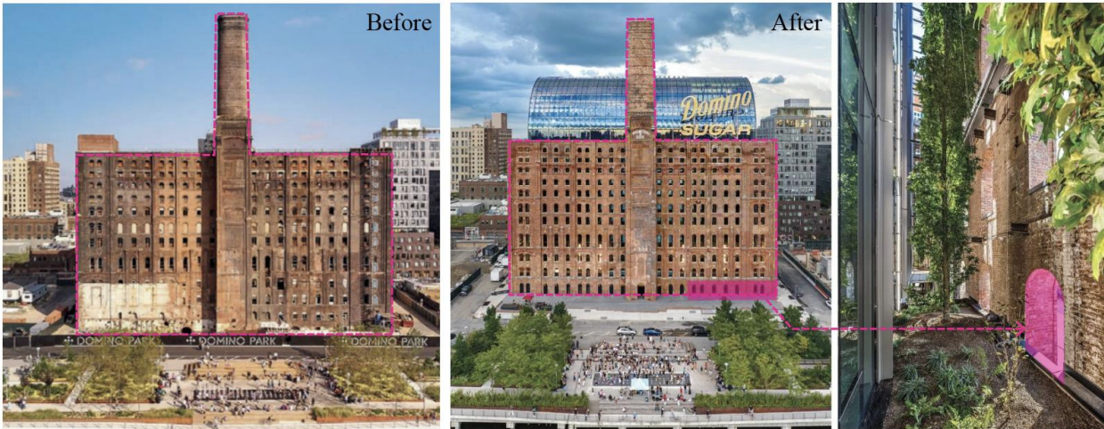
Figure 3-21 Facade texture analysis
