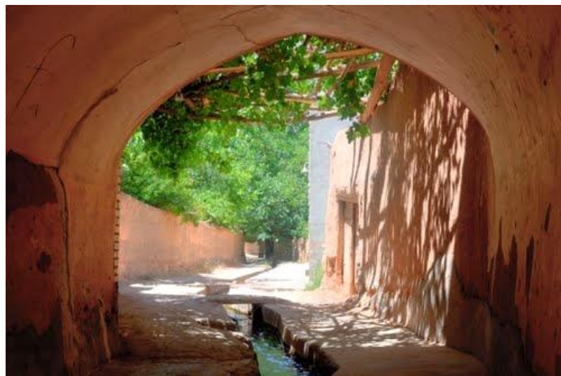
Figure15. Sabat Passageway (a kind of shaded passway with a roof) (Source: https://www.hamshahrionline.ir/news/290135/ )
