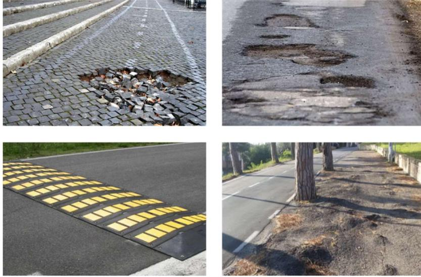
*Figure 1.11. Examples of road surface irregularities that can cause a vibrations to a two-wheeled vehicle*
