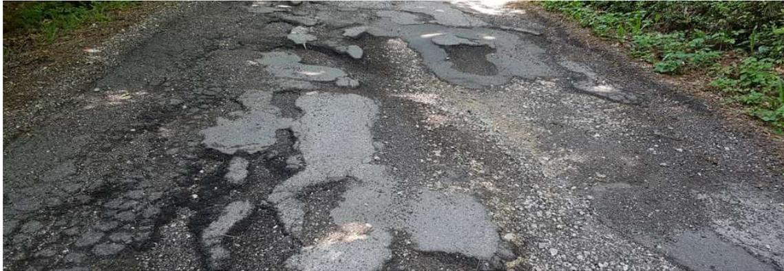
*Figure 3.6. Road surface degraded by potholes*
