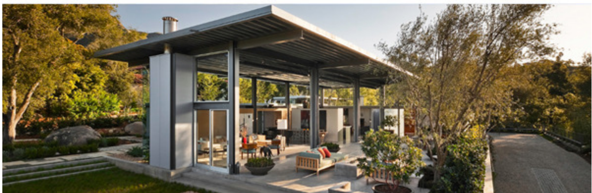
Werner Sobek, House R128, Stuttgart, Germany, 2000.
