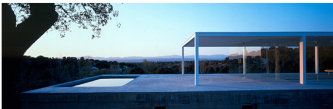
Kengo Kuma, Water/Glass House, Atami, Shizuoka, Giappone, 1995. Alberto Campo Baeza, de Blas House, Sevilla La Nueva, Madrid, Spagna, 2000
