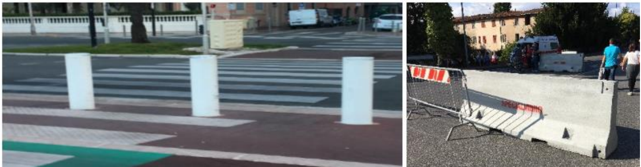
Figure 1.3 – Examples of bollards and temporary re-deployable barriers
