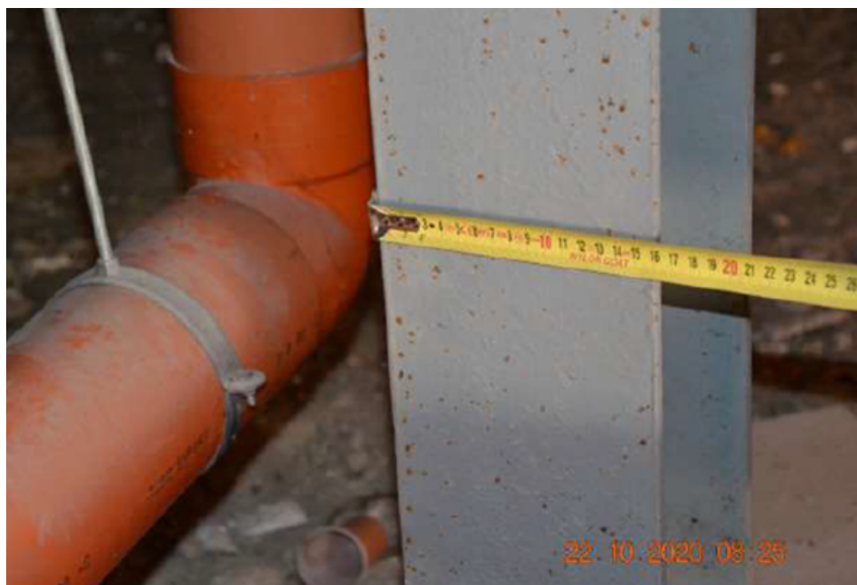
Figure 2.11: shape of a column HEA160 drawn as HEA 180
