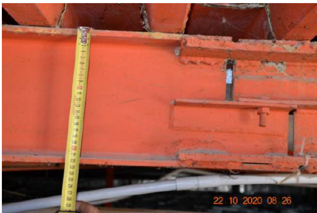
Figure 2.12: Hinged connection at the level of raising floor
