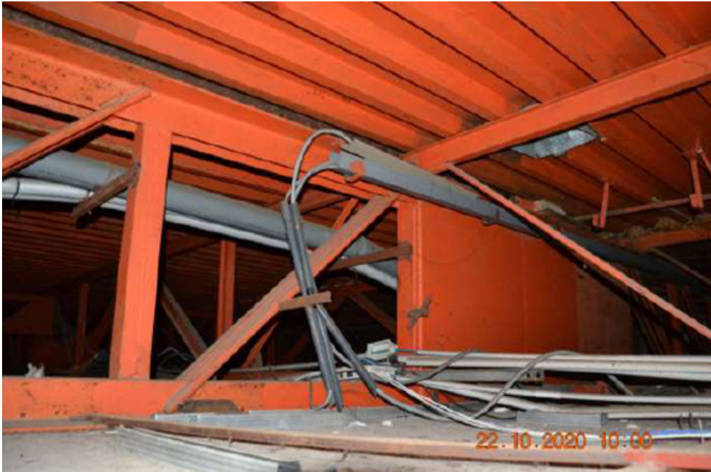
Figure 2.13: Detail of a rigid connection at the truss main beams
