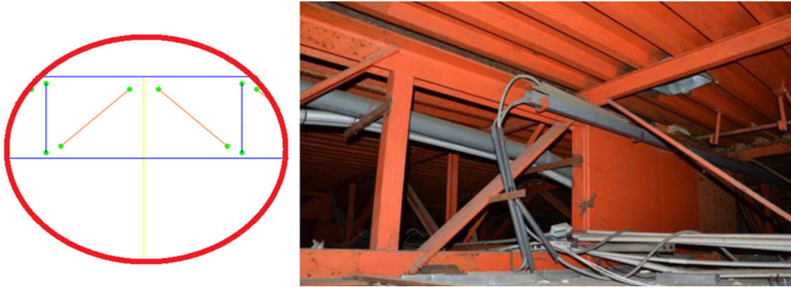
Figure 2.25: scheme of truss beams modelling
