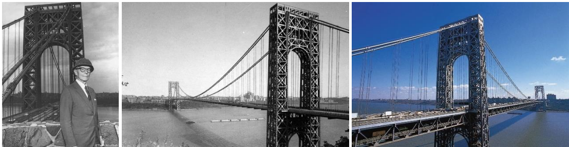
Figure 1-16: (a) O. Ammann [5]; (b) George Washington Bridge 1 st deck conf. (1931) [23]; (c) double truss deck conf. (1962) [24]
