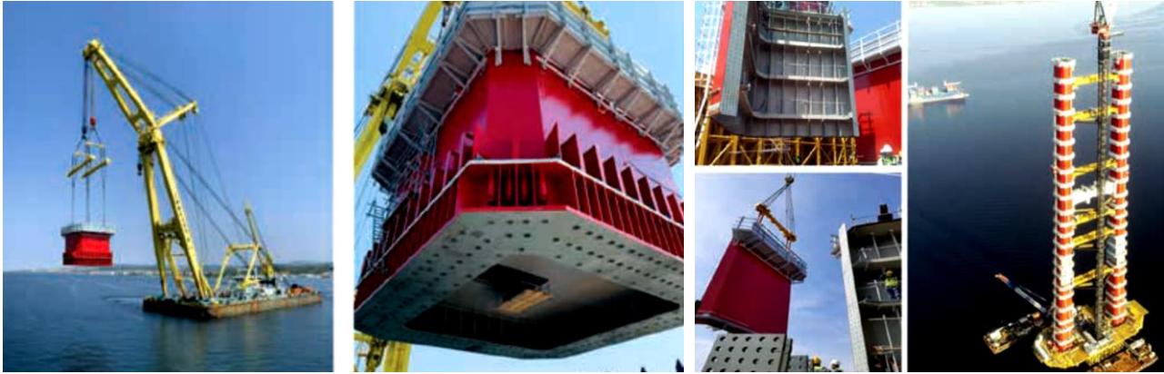
Figure 3-20: Full block lifted by offshore floating crane (left); L-shaped half-block lifted by tower crane (right) [70]
