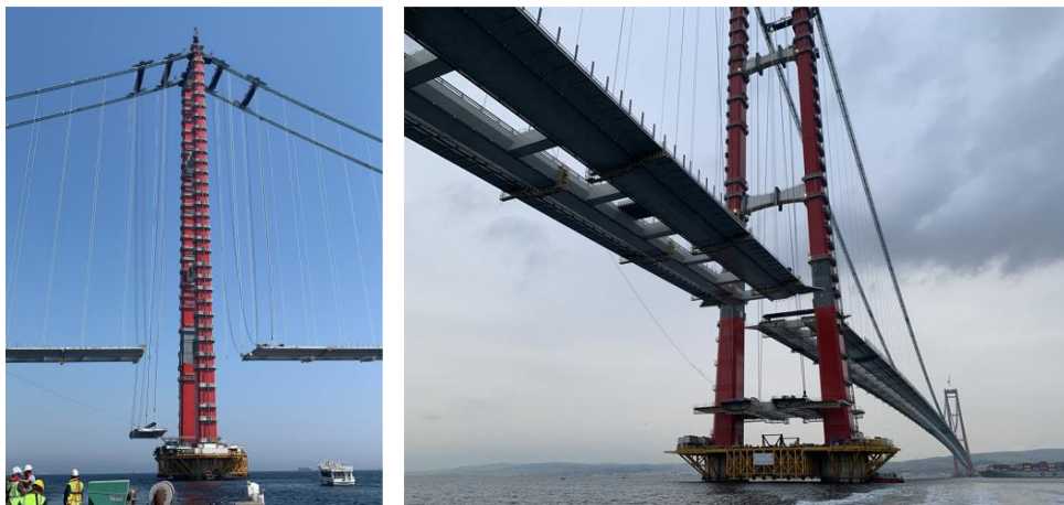
Figure 3-10: Single deck segment lift near the tower (a, left); European tower deck block lift (b, right) [61]
