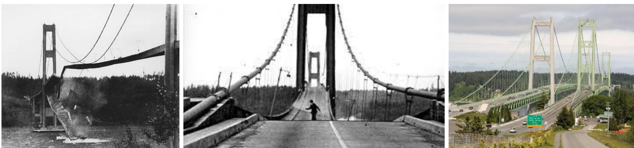
Figure 1-19: Tacoma Narrows Bridge collapse (Moiseiff, 1940) [5]; Modern Tacoma Bridge (opened in 1950 and 2007) [29]
