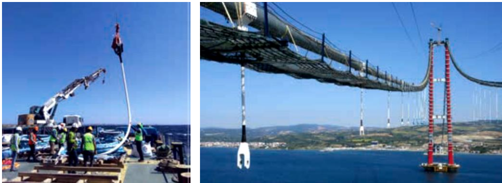
Figure 3-30: Hangers' installation [72]
