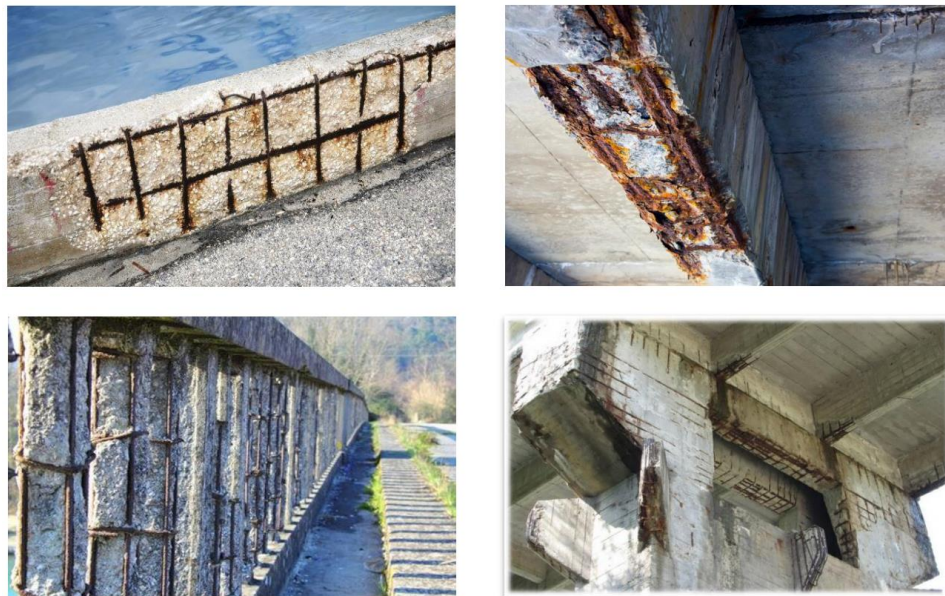
Figure 2: Chloride corrosion steel bars
