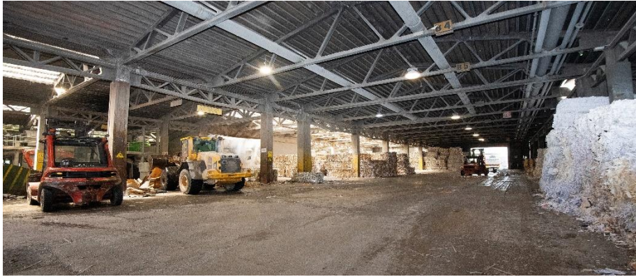
Figure 13: Storage of raw materials
