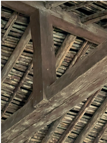
② Central Strut & Correa (Tie Beam) Union
