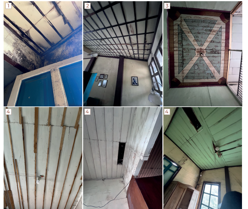
Figure 124: Connections & Elements Decay- Ceilings.
