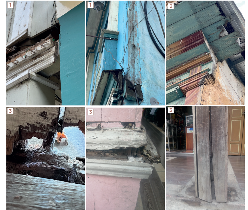
Figure 121: Connections & Elements Decay- Material Crumbling.
