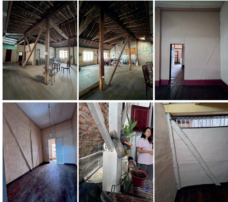
Figure 117: Structural Layout Decay- Distribution of Diagonals.
