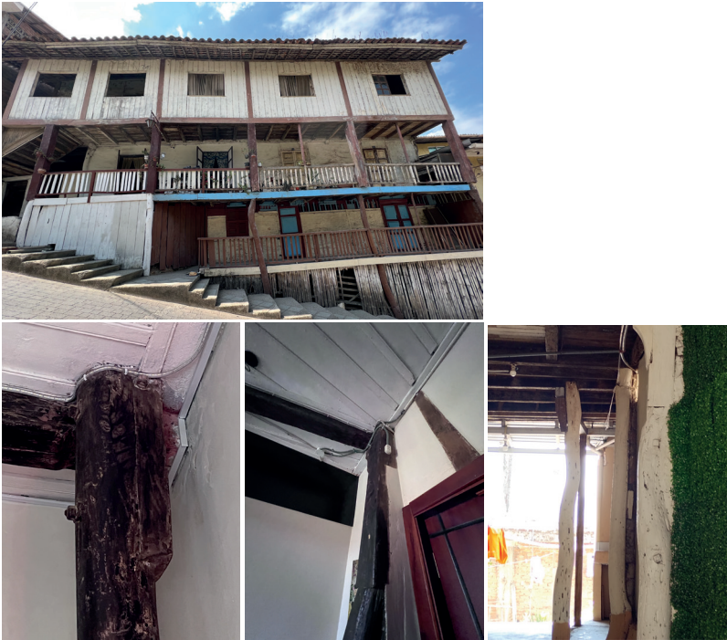
Figure 115: Structural Layout Decay- Warping of vertical elements.
