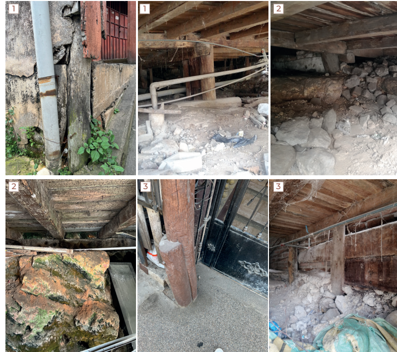
Figure 118: Structural Layout Decay- Foundations Defects.
