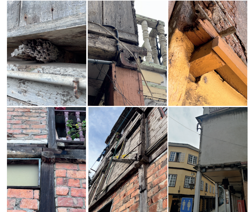
Figure 120: Connections & Elements Decay- Exposed Elements.
