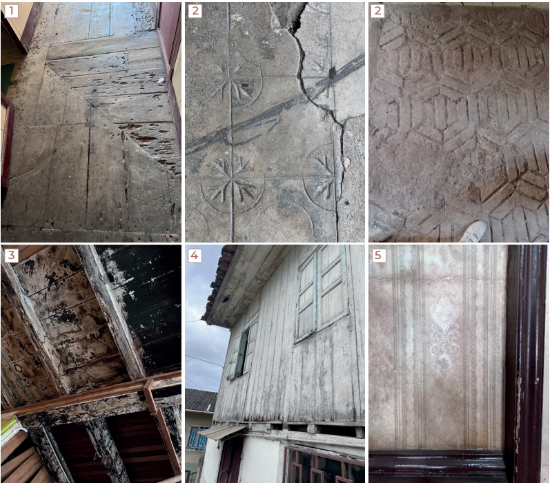
Figure 127: Connections & Elements Decay- Walls and Floors.
