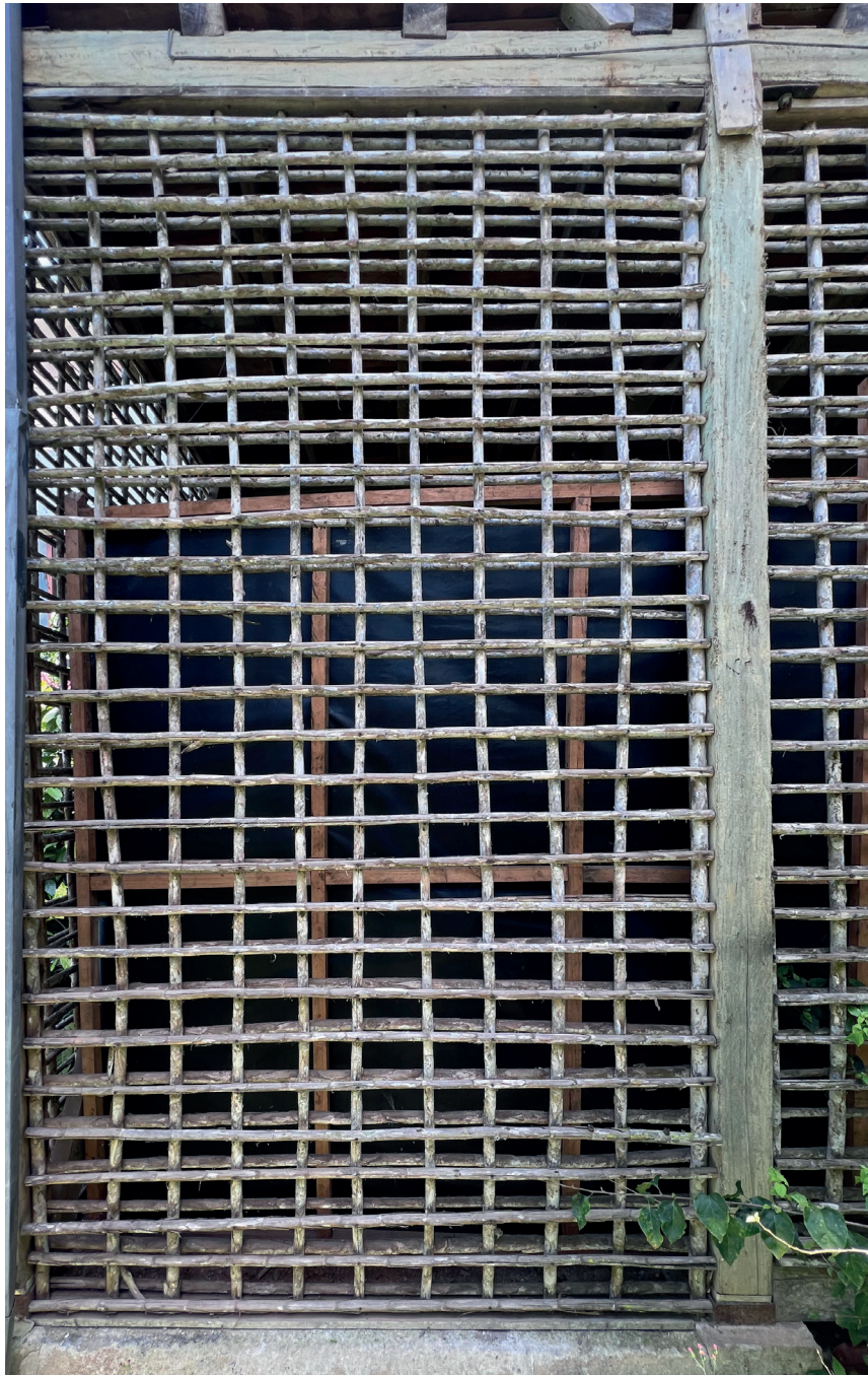
Figure 91: Photographs of bahareque structure.
