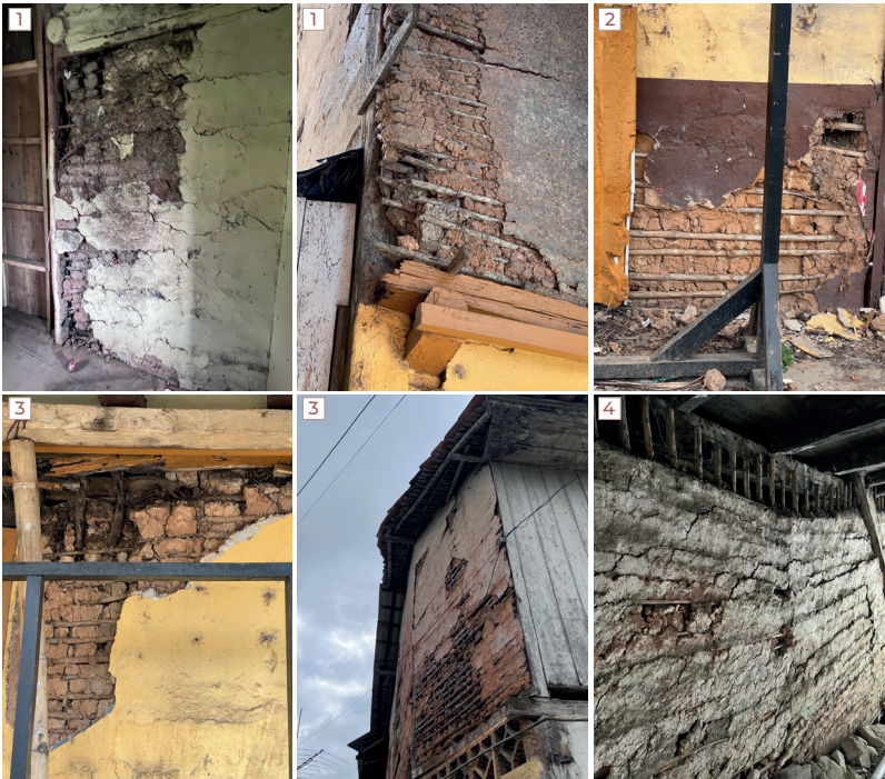
Figure 126: Connections & Elements Decay- Bahareque.
