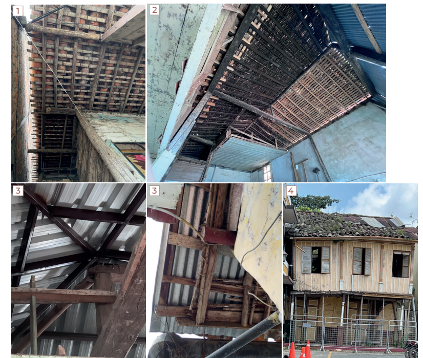
Figure 123: Connections & Elements Decay- Roof Elements.
