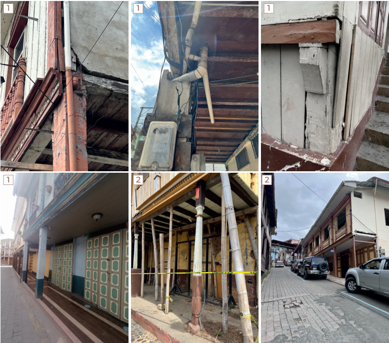
Figure 116: Structural Layout Decay-Replacement of original technique.
