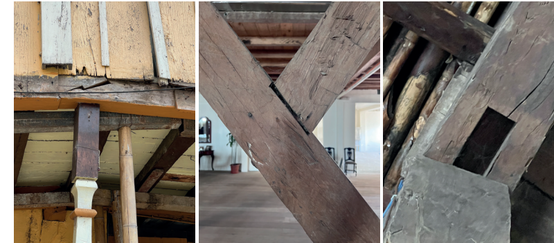
Figure 119: Connections & Elements Decay- Assembly Defects.
