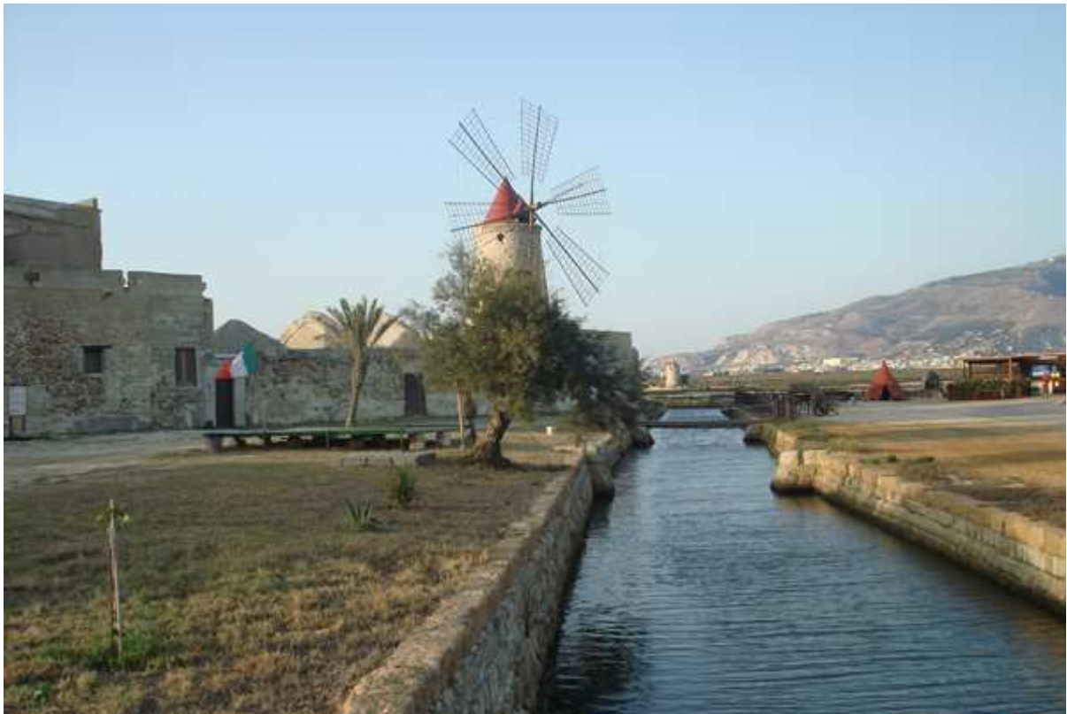
One of the saltworker structures to be recovered, “Case Calcara” of Nubia
