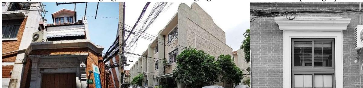
Figure 49 Horizontal and vertical sunshade components Source: Self-photographed
