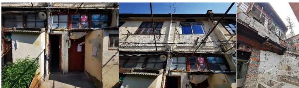
Figure 48 Overhanging blocks and overhanging cornices Source: Self-photographed
