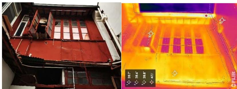
Figure 40 Material of the south-facing facade of sample 1 and thermal imaging on a hot day
