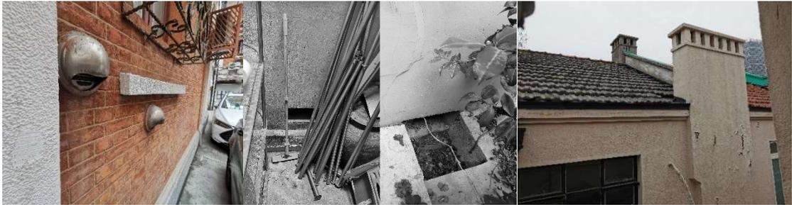
Figure 45 Ventilation holes are opened towards the secondary alley, ventilation holes and chimneys running through the secondary alley-entrance garden-living room-back room-back patio Source: self-photographed
