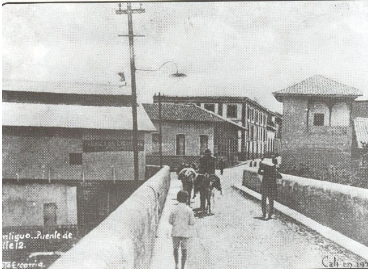
Old Ortíz Bridge on Calle 12, Cali Urban Center, 1920
