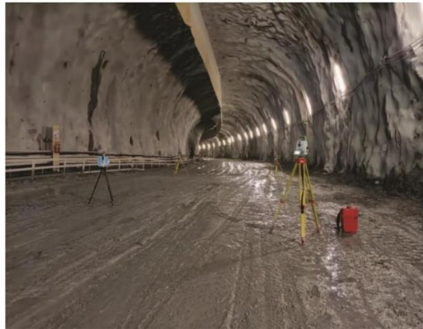
**Figure 2.4 Optical monitoring operation with total station (Bilotta et al., 2022)**
