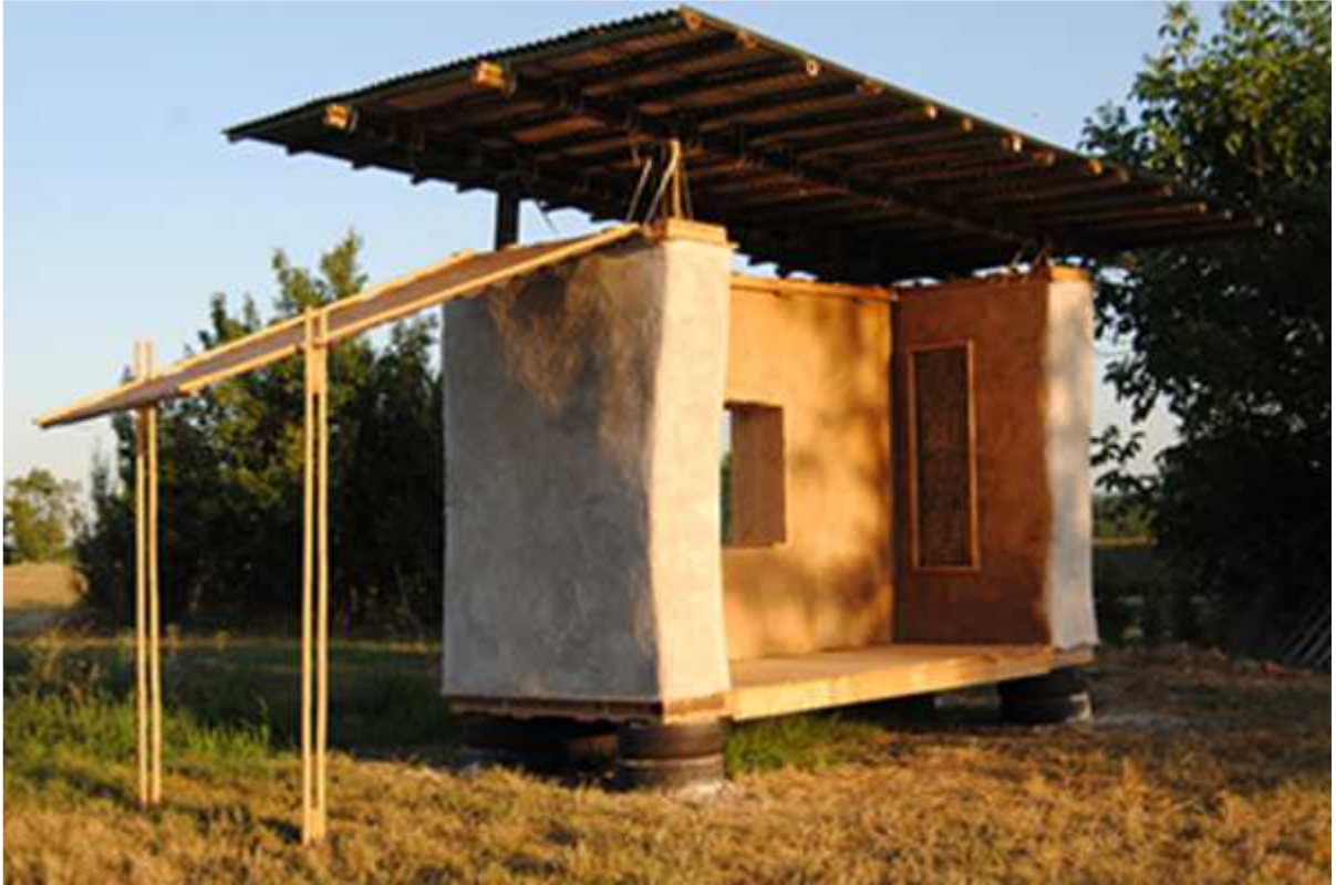
Prototipe scale 1:1 built with straw bale load-bearing realised in Poirino, Torino
