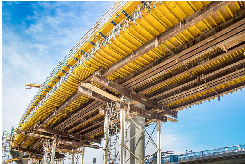
Figure 2.5: Stationary formwork construction method
