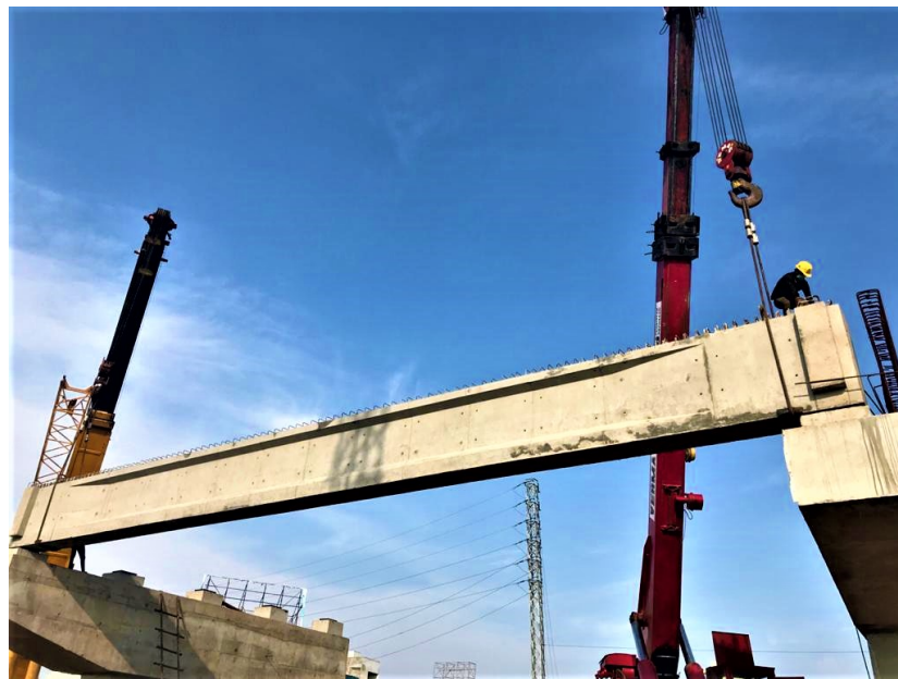
Figure 2.4: Lifting construction method
