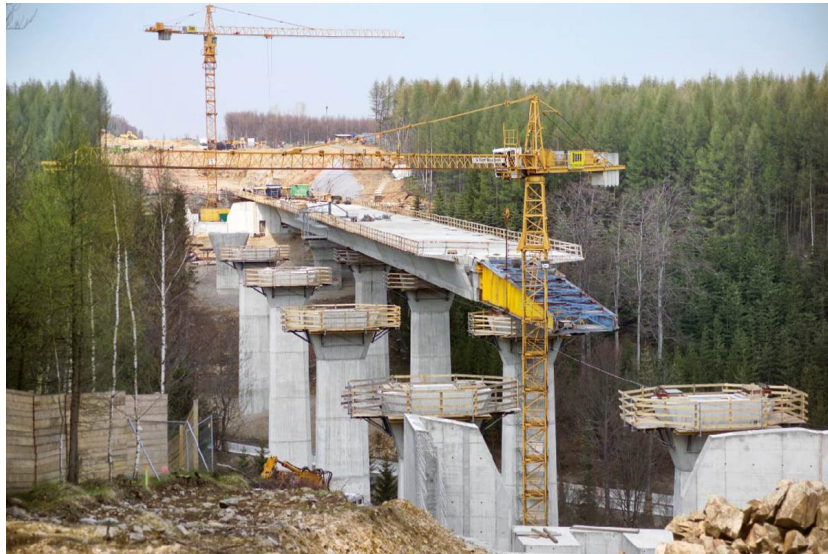
Figure 2.6: Incremental launching construction method
