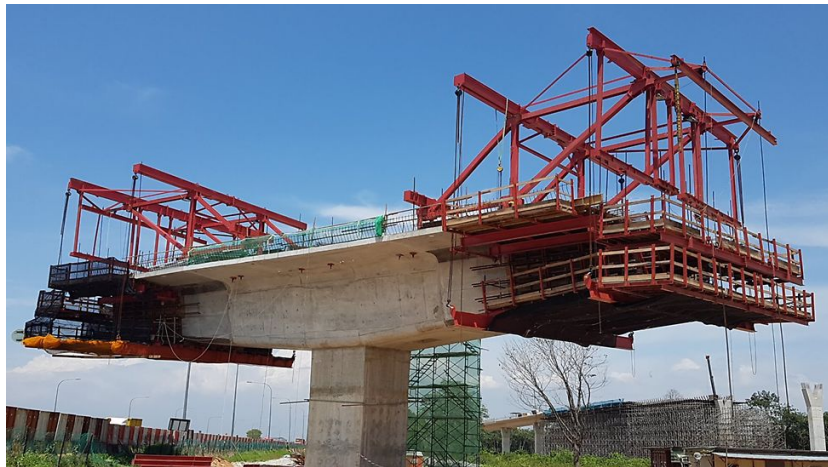
Figure 2.7: Balanced cantilever construction method
