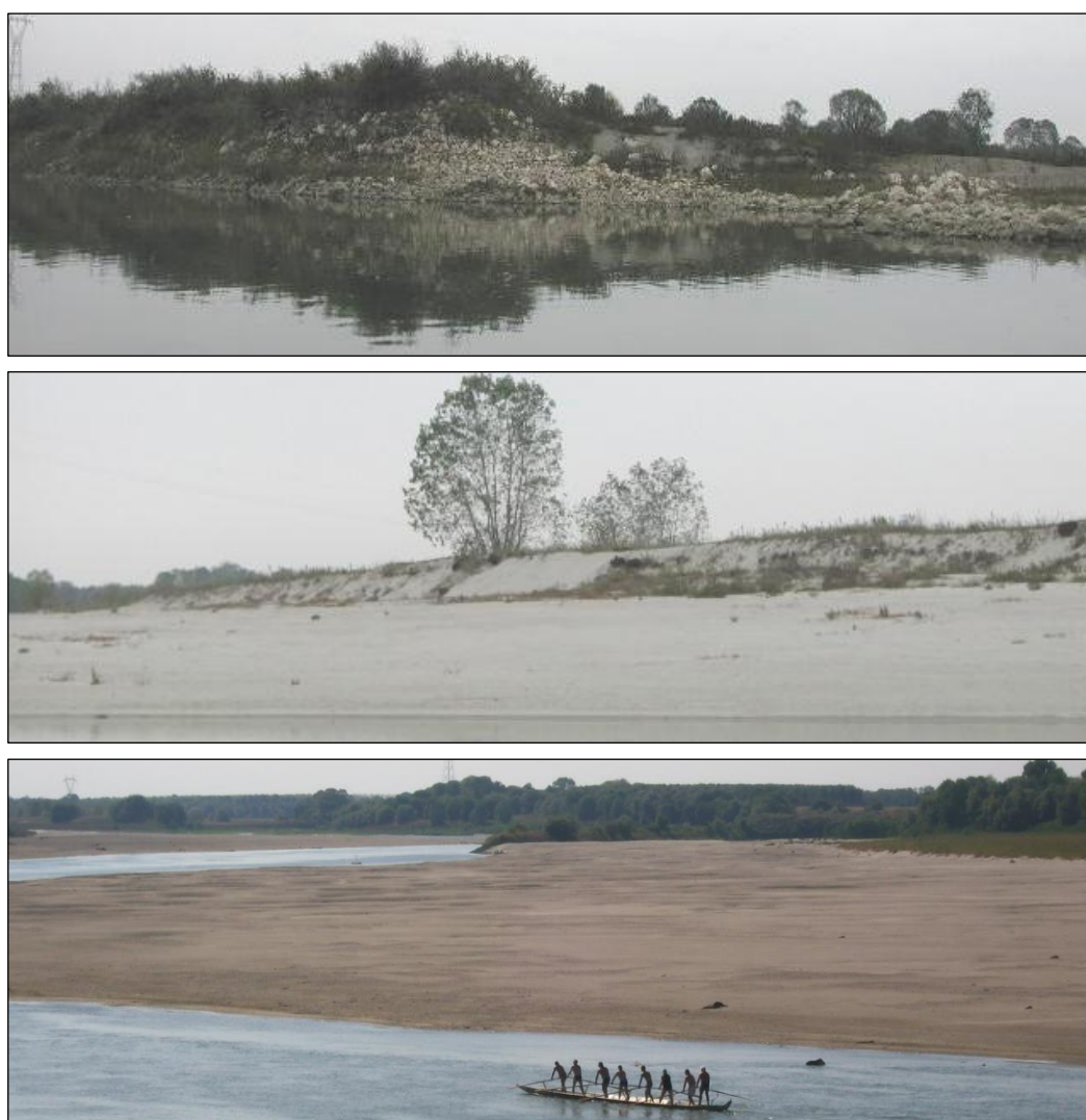
Figure 44. Top: Photo n°159 showing the longitudinal training wall located between progressive 366 and 367; Centre: Photo n°162, depicting bar 616 and 617, namely the depositional area overleaf of the previous longitudinal training wall. This part of the river was in past time an active part of the incised channel (source: ADBPO); Bottom: A picture of the Po River shot from the section just downstream of the conjunction between the tailrace and the meander loop. It is possible to appreciate the extent of the point bar located on the hydraulic left at the conjunction mainly generated by the upstream longitudinal training wall (source: Google Earth).
