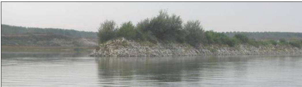
Figure A - 6: Photo n°161 and Photo n°163 revealing the longitudinal training walls.
