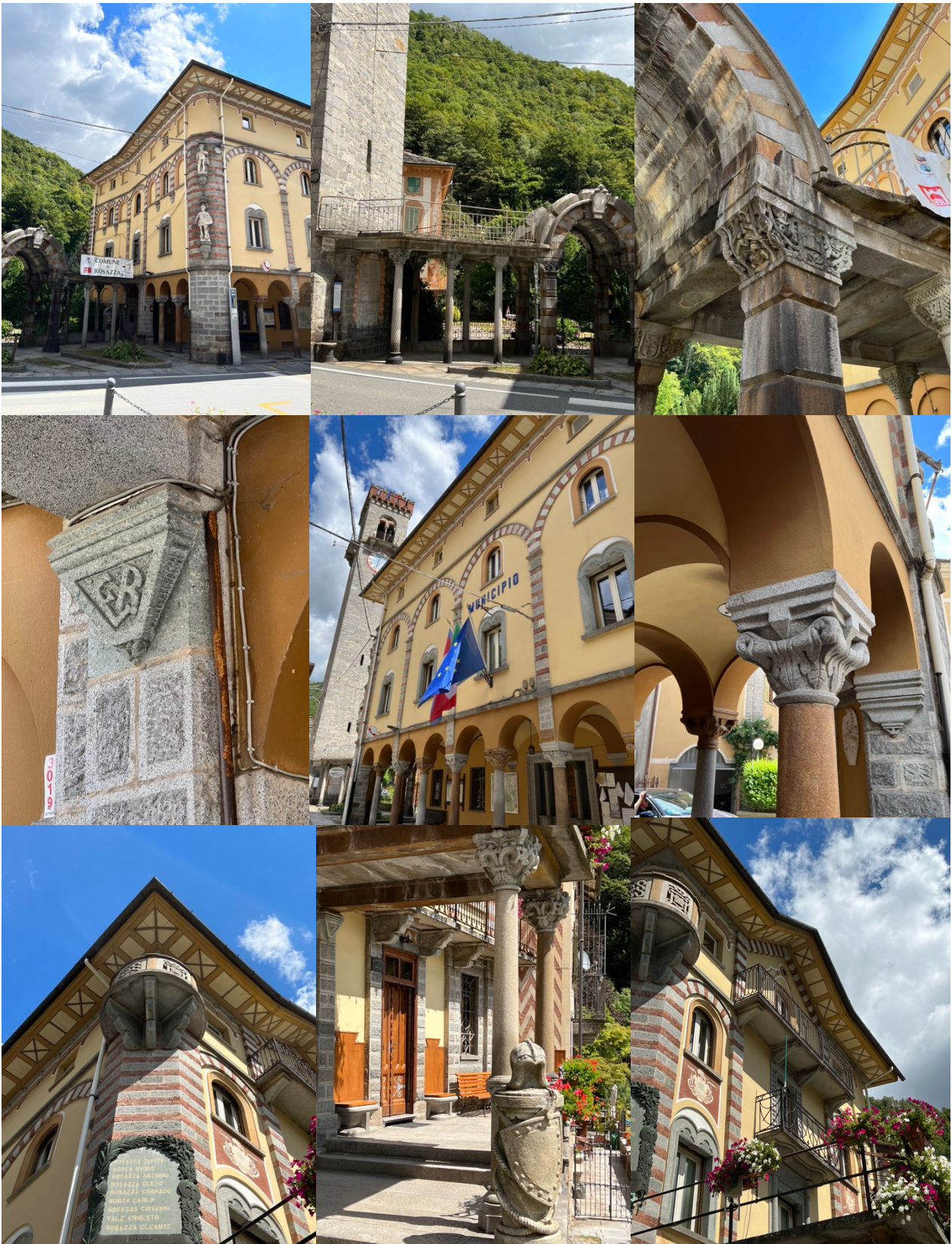
Figure 16 City Hall of Rosazza, also known as La Palazzina. Richly decorated building designed by Maffei in perfect Eclectic style, shows the refined stone decorations that determine the whole town's aesthetic (Personal photographs).
