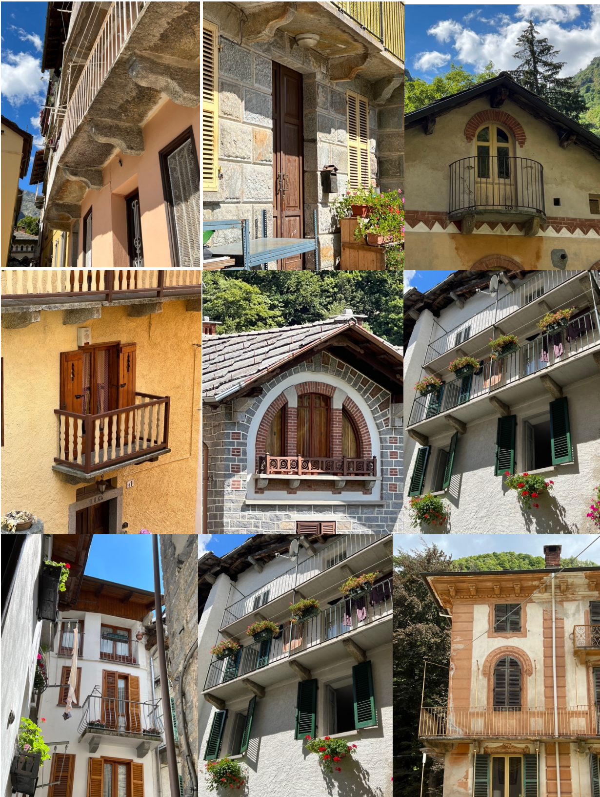
Figure 12 Examples of balconies in the town. It is evident how the typical stone of the valley, syenite, was used in every construction detail. (Personal photographs)
