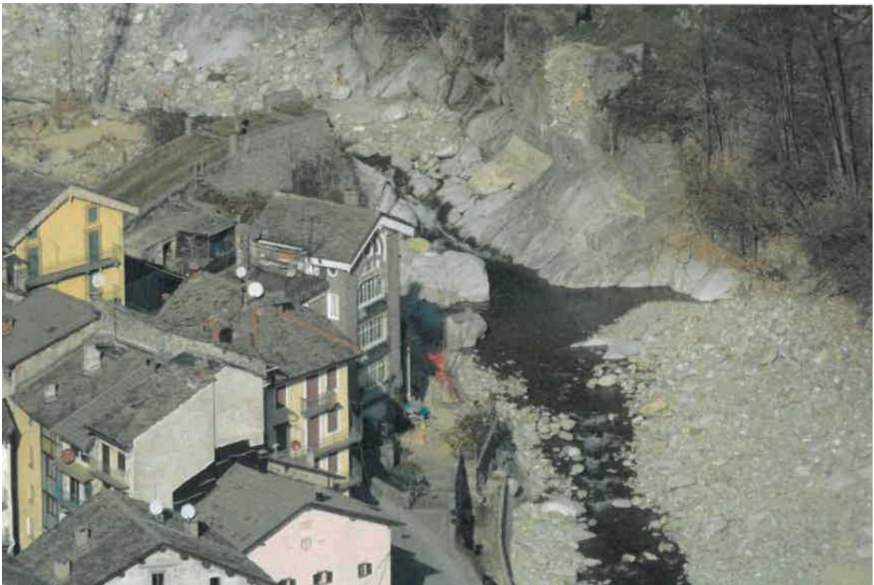
Figure 34 Valz Blin's building after 2020 flood. It is visible how the house was hit by the flood and possibly by the fall of Ponte delle Cave. (Valz Blin, 2022)
