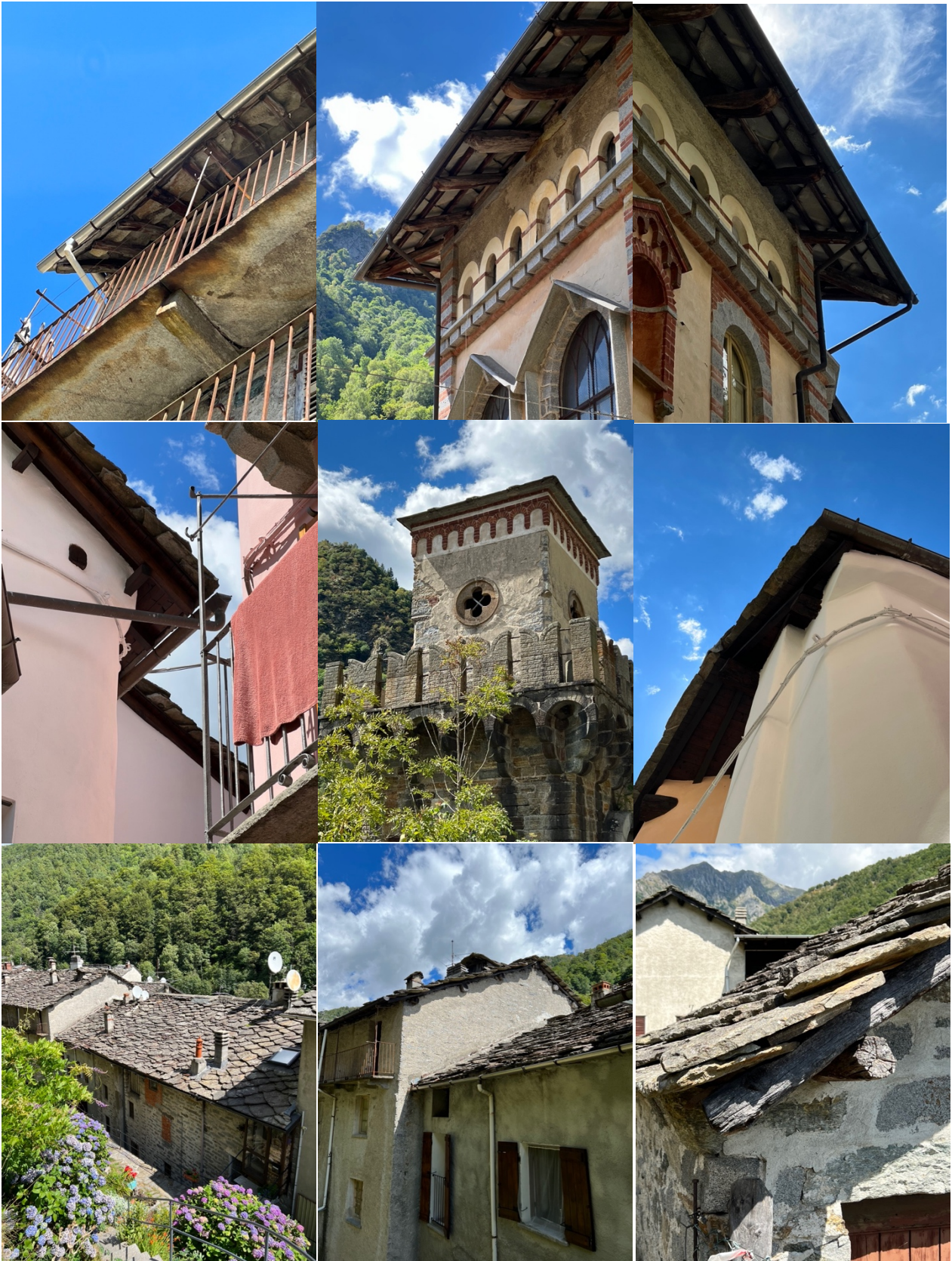
Figure 13 Examples of roofs in buildings of Rosazza. It is possible to see how generally the roof typology is a wooden structure with stone panels on top. (Personal photographs).
