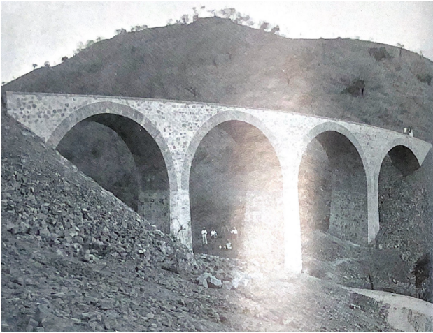
Figure 10 Railway bridge of Saati-Ghinda (Eritrea) - year 1902.
