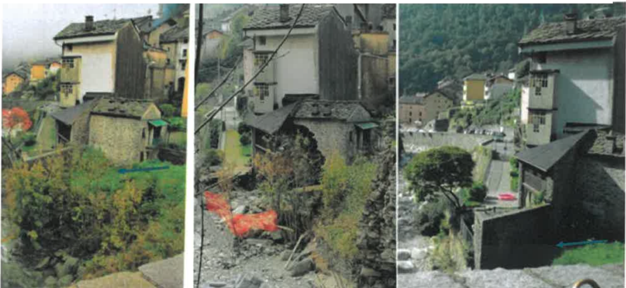
Figure 35 Damage to Valz Blin's building. (Valz Blin, 2022)
