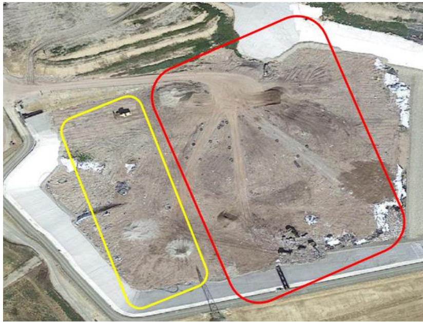
Figure 43 - Active part of the landfill.
