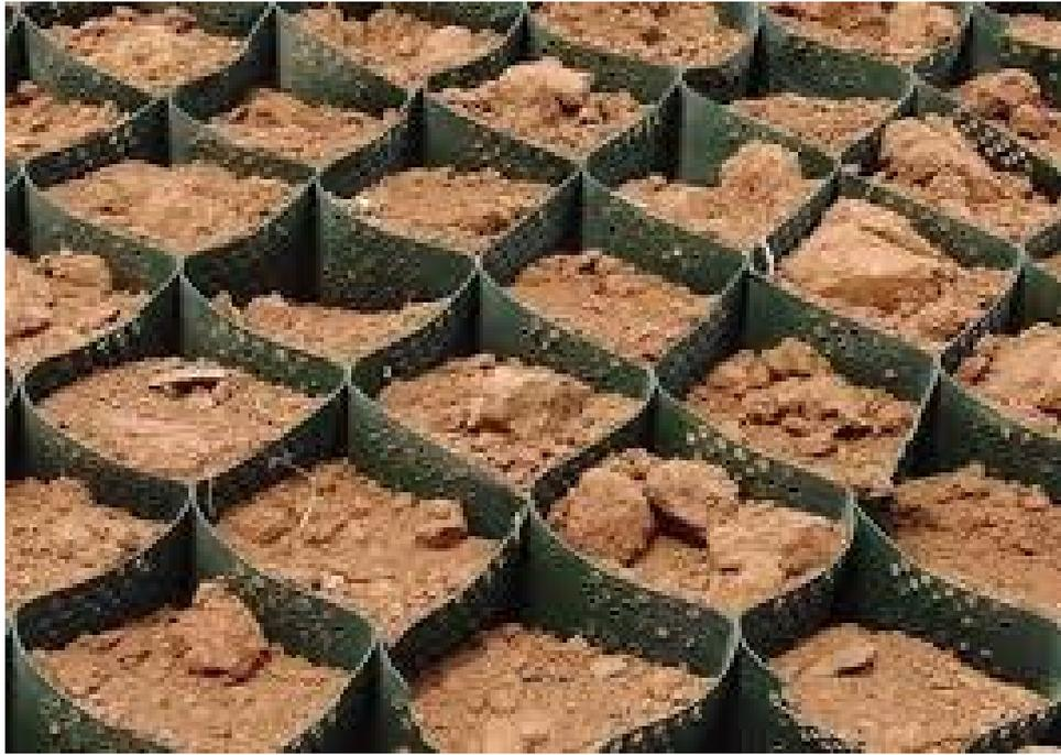
*Fig. 8 - Geocells filled with granular soil*
