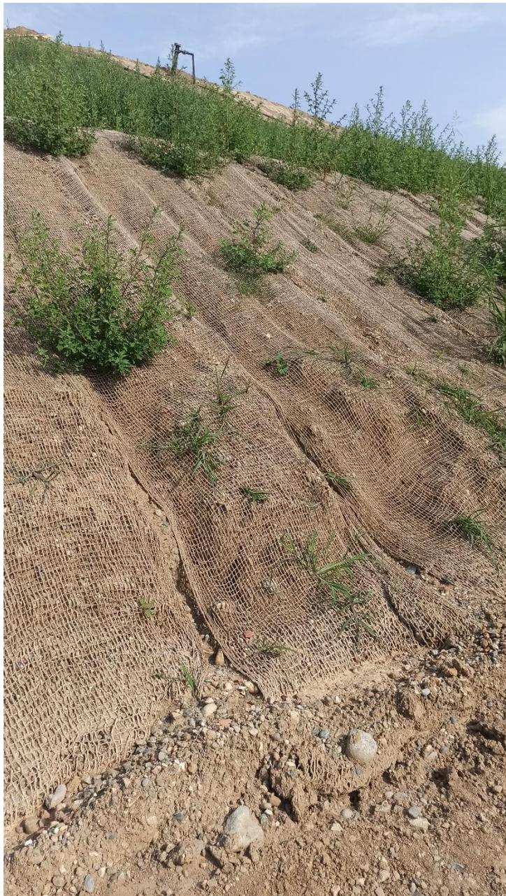
*Fig. 63 - Use of geosynthetics to promote slope greening (Oggeri and Capozzo, 2022)*
