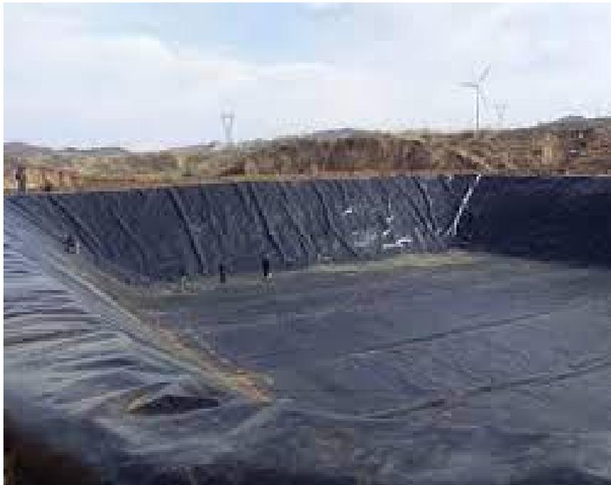
*Fig. 5 - Use of geomembrane for base lining of a landfill site*
