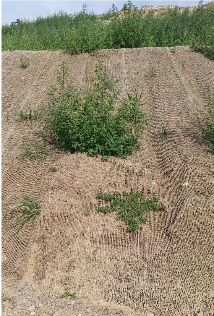
*Fig. 1 - Use of geosynthetics to prevent slope erosion (Oggeri and Capozzo, 2022)*
