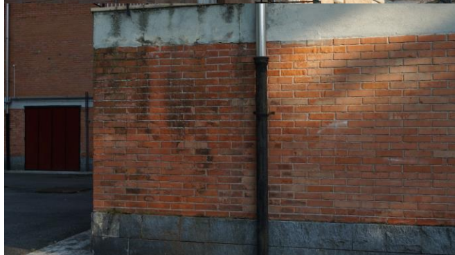
Figure 43. Moldy wall of building
