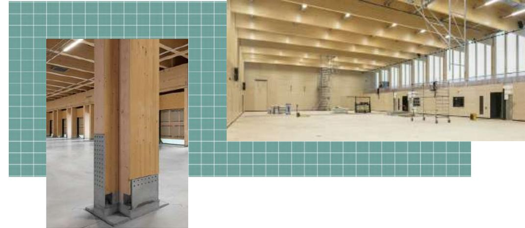
Glue-laminated timber is a structural engineered wood product also within the category of wet systems (glued) that is typically used in applications for beams and columns, its stronger than steel and has more strength and stiffness than comparable sized dimensional lumber (WoodWorks, 2021).
