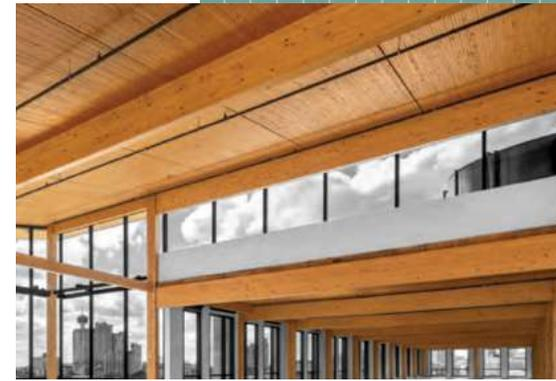
On the other hand one the products within the category of dry systems (non-glued) is the DLT panels. They are constructed from solid sawn timber that is orientated on edge, but the particular thing, as shown in (Fig. 33) is that is friction-fit together using hardwood dowels (WoodWorks, 2021).
